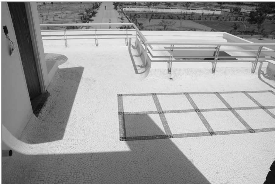
Picture 7: Exposed roof area covered with china mosaic
