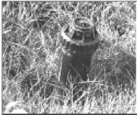
Picture 13: Sprinklers for irrigation
