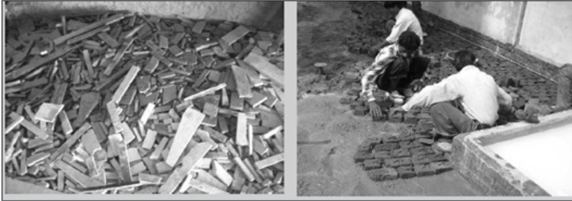
Picture 29: Picture of tile scrap & broken bricks being used for brickbat coba
