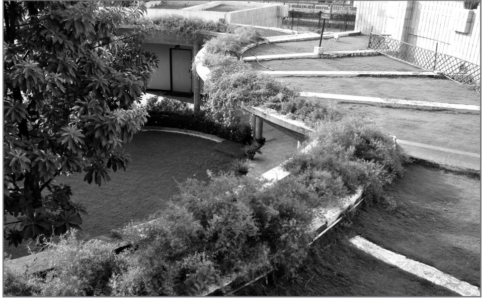
Picture 8: Vegetated roof
